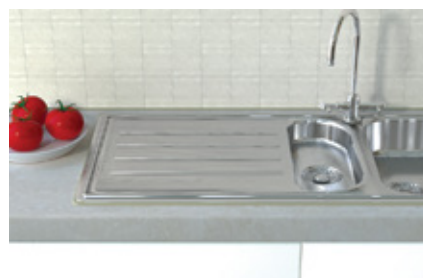
Sealings in the kitchen
