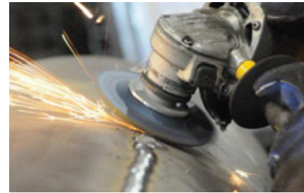
Weld Stock Removal
