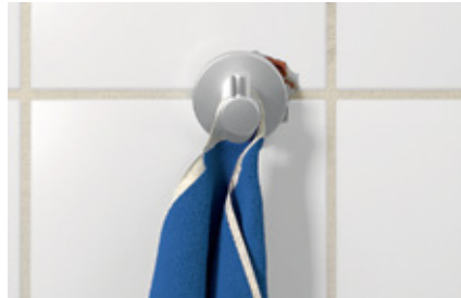
Repairing damaged drill holes
