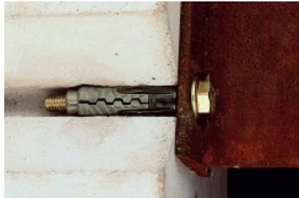
Beam Fixing
