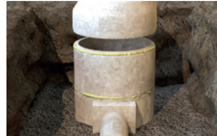
Sealing concrete manhole rings
