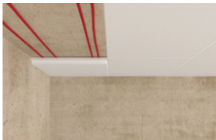
Insulation panels on the ceiling
