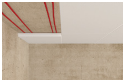
Insulation panels on the ceiling
