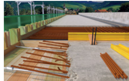
Rebar connections
