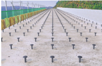
Upgrade of bridges
