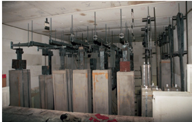
Before the fire test
