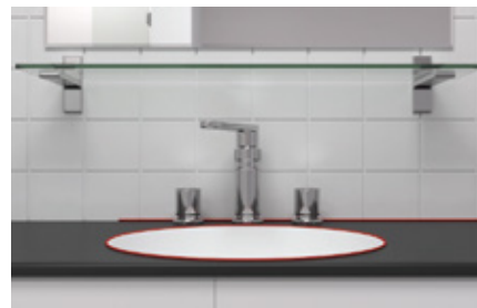
Sanitary joints at washbasins
