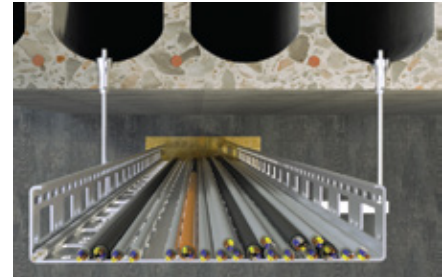
Cable trays in pre-stressed hollow-core concrete
