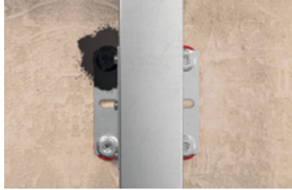
Sealing of the screw heads
