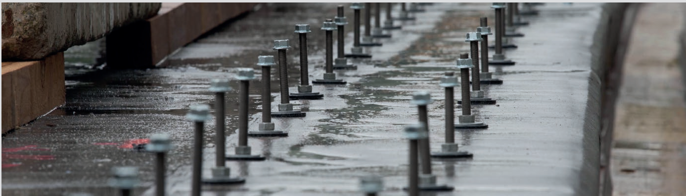
Bridge edge beam fixing
