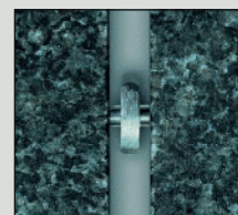
Appearance of joint with conventional dowel fixing
