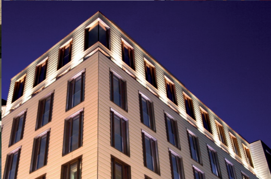
Neuer Wall 52, Hamburg. Glass shingle façade, fixed with FZP-G on SystemOne light.
